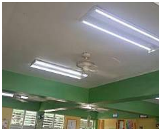
FIGURE 15: INSTALLATION OF ENERGY EFFICIENT LIGHTING
