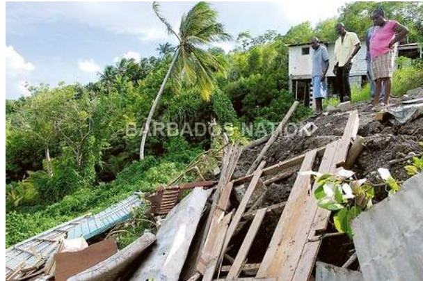
FIGURE 3: RESIDENTS LOOKING AT THE MANGLED HOUSE WHICH COLLAPSED AS A RESULT OF THE INSTABILITY OF THE LAND.
